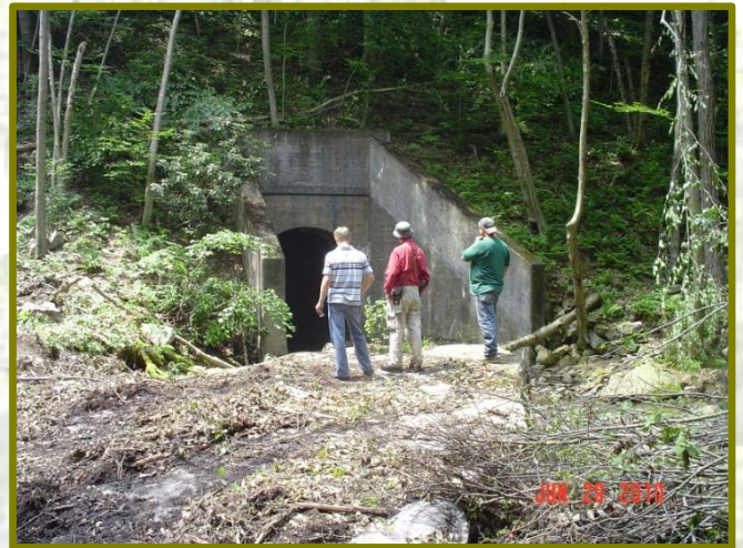
BOFDAC staff evaluate options for the 100-year-old Jonathan Run horseshoe arch culvert
