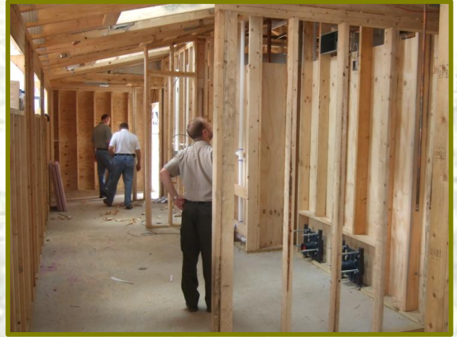
FDC-414-961 - Promised Land State Park Pickrel Point & Deerfield Campground Rehabilitation Inspection of the framing and rough-in work
