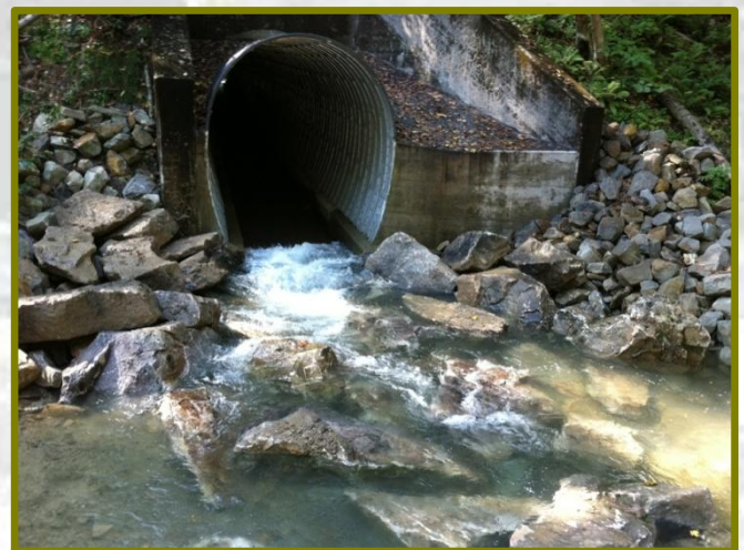
Completed rehabilitation of the horseshoe arch culvert – Jonathan Run under the Great Allegheny Passage Rail Trail
