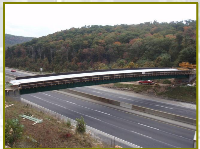
LHHT Bridge – Single span structure, spanning the PA Turnpike, Somerset County
