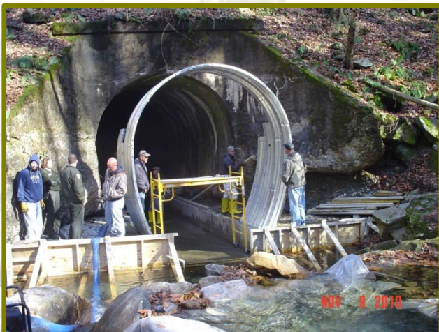
Initial alignment, assembly and installation of the galvanized steel liner system
