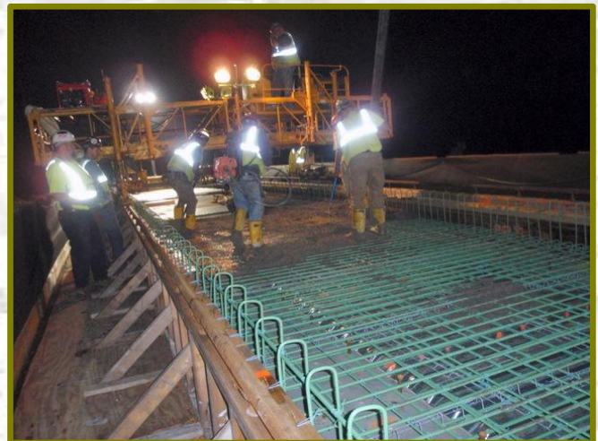
FDC-219-2239 - Laurel Ridge State Park Laurel Highlands Hiking Trail Bridge Placing and screeding the concrete deck
