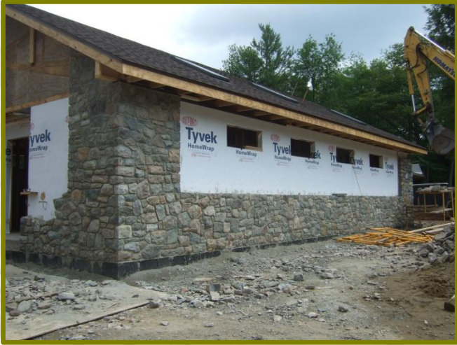
FDC-414-961 - Promised Land State Park Pickrel Point & Deerfield Campground Rehabilitation Installation of stone veneer - Pickrel Point Wash House
