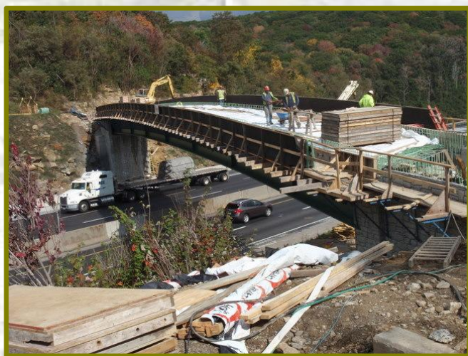
LHHT Bridge – Construction continues to progress with placement of parapet walls and deck
