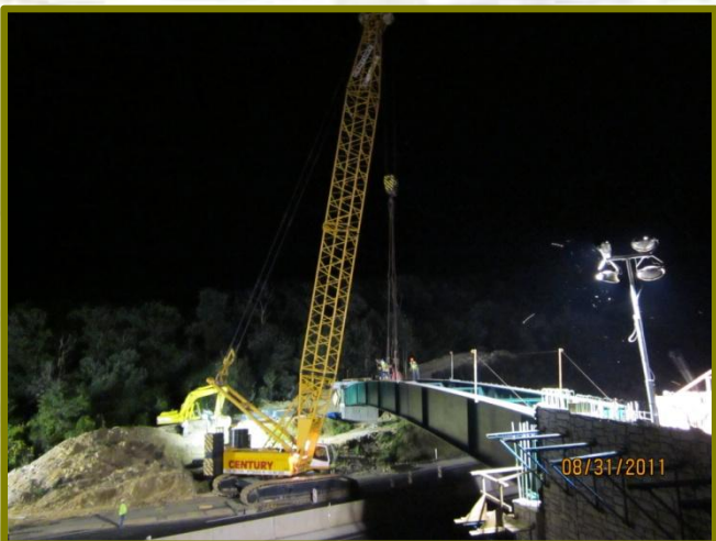
FDC-219-2239 - Laurel Ridge State Park Laurel Highlands Hiking Trail Bridge A crane setting the single span, steel superstructure across the turnpike
