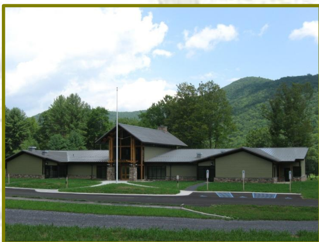
The new Wildlife Center at Sinnemahoning Sinnemahoning State Park
