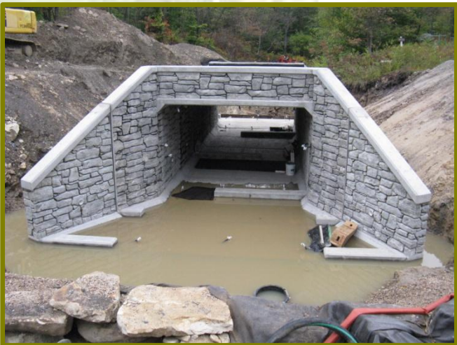
FDC-006-6476 - Gallitzin State Forest Structure Replacement Bridge No. 06-0004 Placement of reinforced, precast concrete box culvert sections
