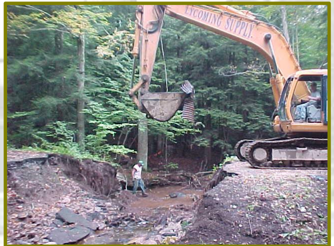
FDC-020-7182 - Loyalsock State Forest Structure Replacement Bridge No. 20-9011 Demolition of existing CM pipe structure & excavation for new box culvert construction
